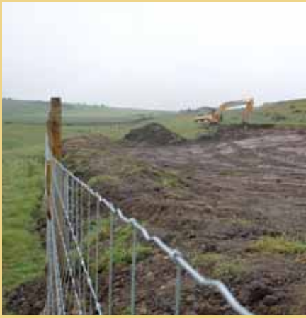
Work in progress on the coastal site.
