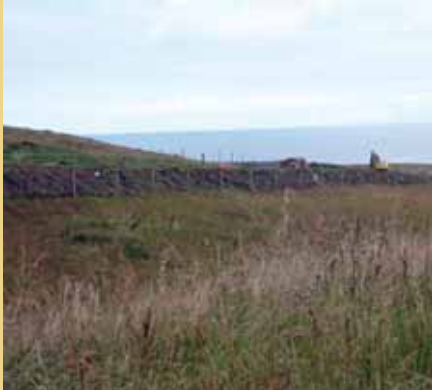
Work commences on the site for the pipeline.
