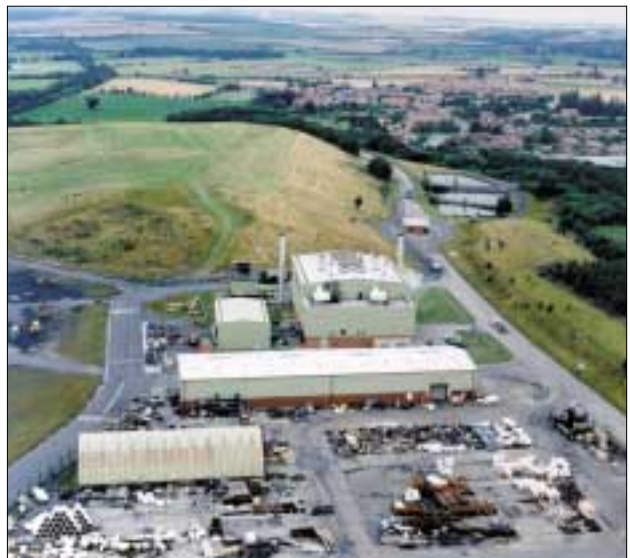
Figure 11. Harworth CHP plant (courtesy of UK Coal Mining Ltd)
