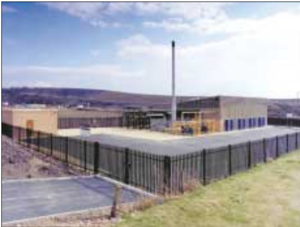
Figure 2. 5MW e AMM power plant at Hickleton, UK (courtesy of Octagon Energy Ltd)
