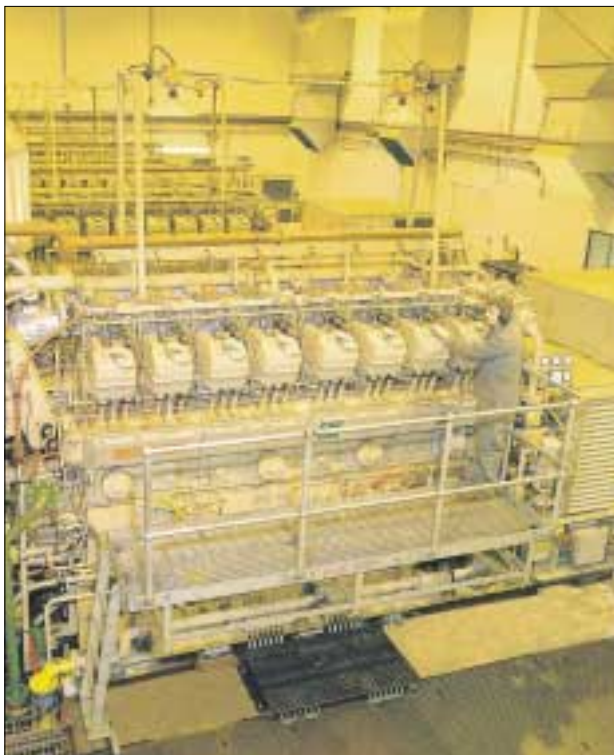
Figure 8. Spark-ignited gas engine (courtesy of MAN B&W Diesel Ltd)
