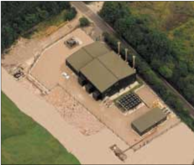
Figure 12. Bentinck Generating Station (courtesy of Warwick Energy Ltd)
